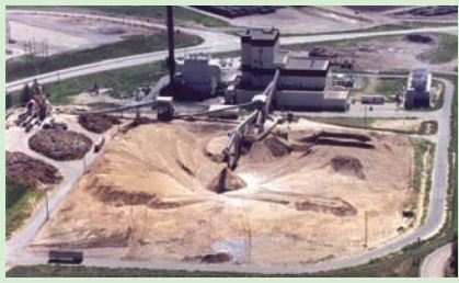
Williams Lake Generating Station has been generating electricity from biomass continually for over 15 years.
